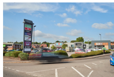
Southampton Road Retail Park, Salisbury
