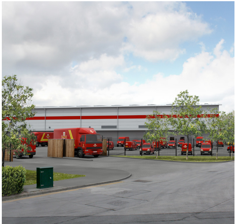
1-2 Auriol Drive & Carr Road, Greenford
